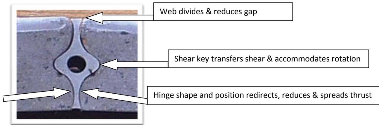
TripStop™ in partially uplifted slabs (In larger uplifts the web tends to move to one side rather than remain central as shown here)
