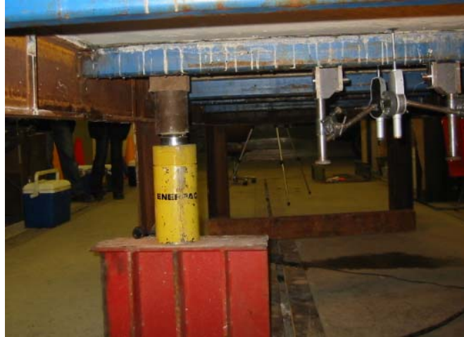
Figure 7. Slab 2 being pushed up at a corner (at point D)
